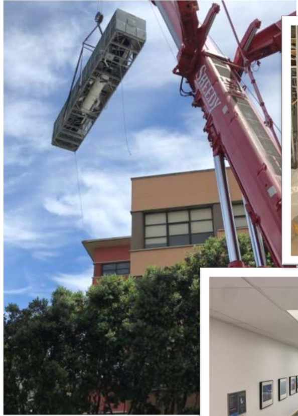
New Long OR Fan being lifted to roof of ED
