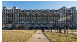
Cook County Hospital Market Rate Redevelopment Illinois, USA
