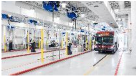
Stoney CNG Bus Storage & Transit Facility Alberta, Canada
