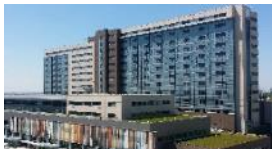
Humber River Hospital Ontario, Canada
